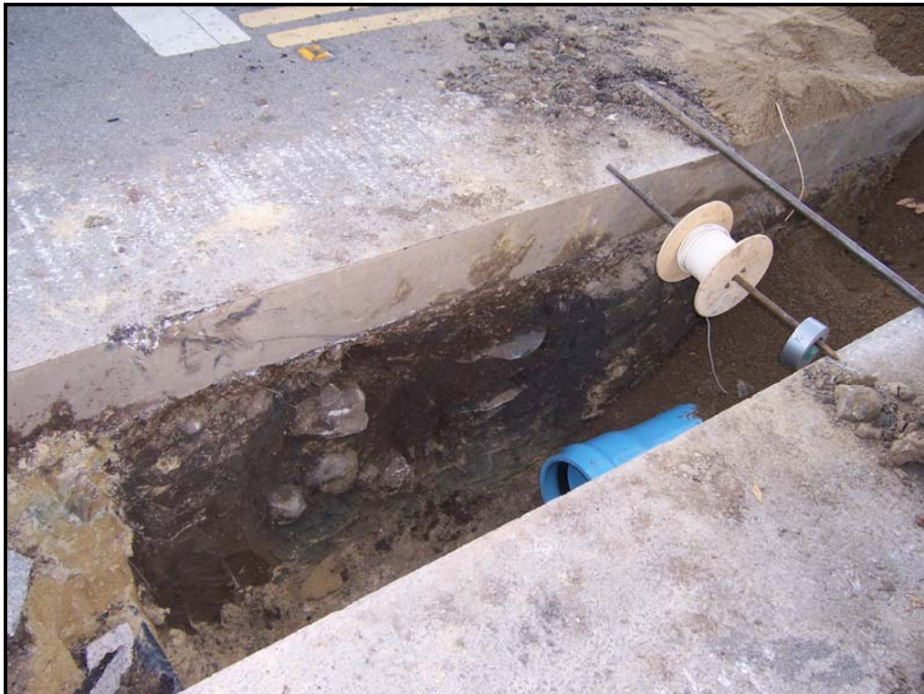
Downtown San Luis Obispo archaeological site uncovered during trenching for utilities, 2005
