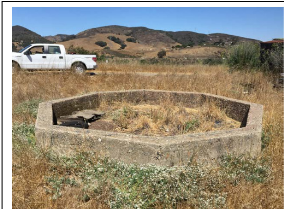
P-40-038310, a 16 to 17-foot wide octagonal silo footing, was identified within the Buckley Road Extension site.
