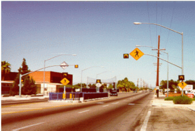
Figure 40. Fences or railings in the median direct pedestrians to the right and may reduce pedestrian crashes on the second half of the street.
