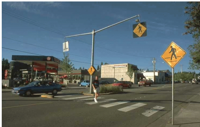
Figure 39. Pedestrian warning signs sometimes are used to supplement crosswalks.
