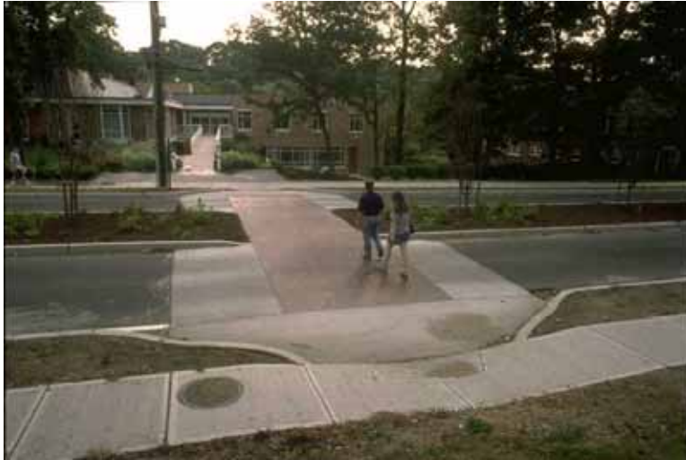
Figure 36. Raised crosswalks can control vehicle speeds on local streets at pedestrian crossings.
