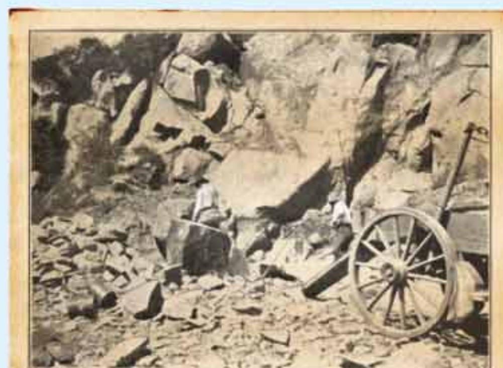
The smaller mines were simple operations: blasting, hand-digging, and hauling broken ore to the railroad.
