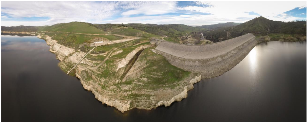
Nacimiento Reservoir Dam, February 2015. Photo credit: County of San Luis Obispo.
