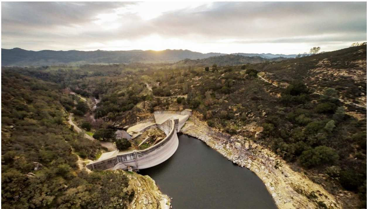
Salinas Reservoir Dam, February 2015. Photo credit: County of San Luis Obispo.
