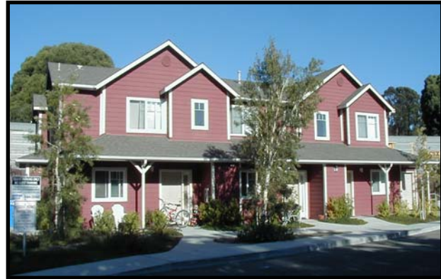
Pismo Street Station Family Housing
